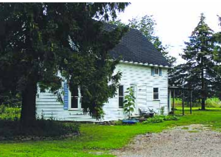
The Gilliam family's first home—a 900-square-foot, two-bedroom, 120-year-old farmhouse—was demolished because of toxic mold.
