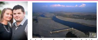
The picture is a picture of the Choulteca Bridge in Honduras. The bridge was engineered to withstand a category 5 hurricane. In 1998, Hurricane Mitch slammed into Honduras and the engineering proved correct. The bridge still stood. But, do you notice a problem with the picture above? Hurricane Mitch was so forceful the river moved! The bridge was perfectly built, but
